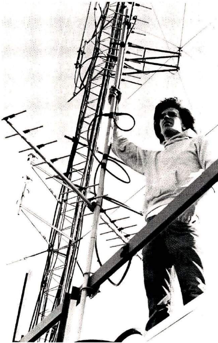
Bill Melody, WA6YBD, takes a moment from antenna work to enjoy the view from the WR6AZA ATV repeater site.
