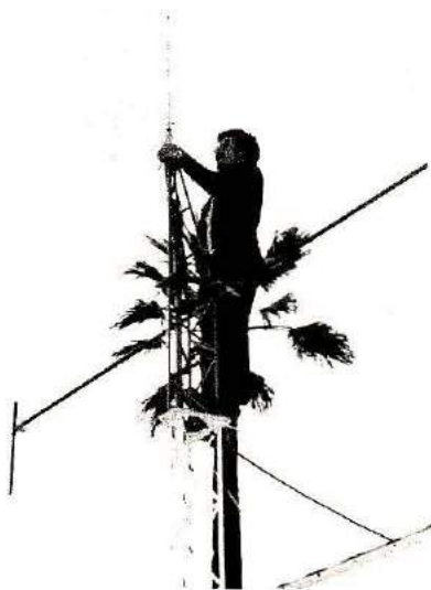
Part of the preparation for the parade includes putting up antennas and checking out the system. Here Wayne Maynard, WB6BFN, is installing a 2-meter antenna atop a temporary tower to provide better reception of the hand-held units (photo by K6PGX).
